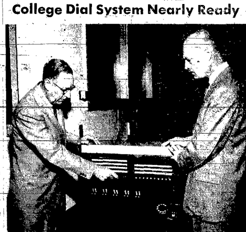
INSTALLATION OF A NEW DIAL phone system on the WSTC campus is expected to be completed next week. Northwest Bell Manager W. G. Schulz is pictured at left above explaining switchboard details to College President W. A. Brandenburg...
